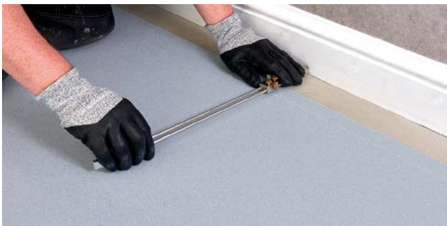
Figure 11 Scribing the wall profile
