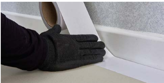
Figure 12 Use double sided Polyflor recommended tape
