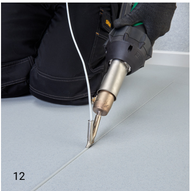
12 Geotone QuickLay can be hot welded at the seams and to coved skirtings upon immediate completion of the installation.
