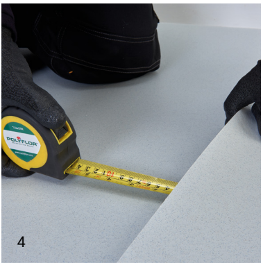
4 Use the appropriate method to install Geotone QuickLay in the room. Allow a 25mm overlap at the seams and cut in to form a tight seam.
